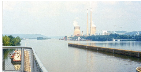
Pleasants Power Station
