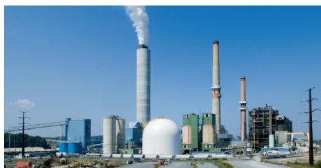
Brunner Island power plant | Talen Energy
